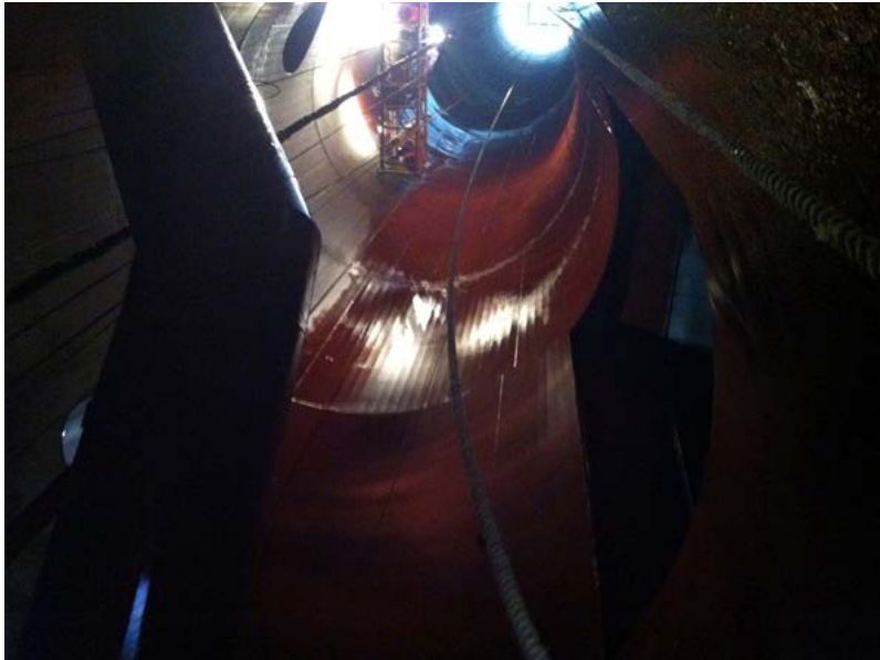
Corr-Paint™ CP2050-LF coats flare stack.
