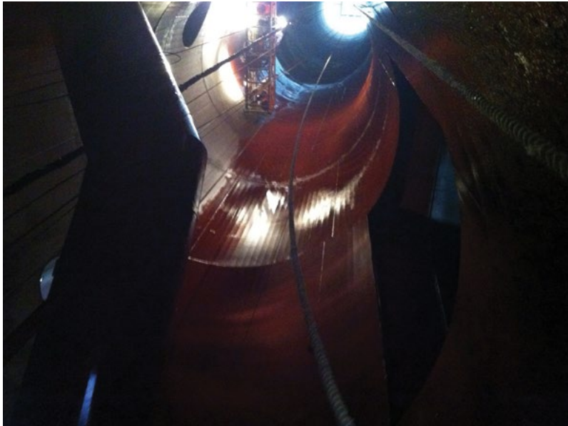
Corr-Paint™ CP2050-LF coats flare stack.
