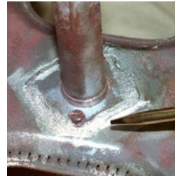
Pyro-Putty® 653 seals corroded burner manifold.
