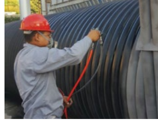
HiE-Coat™ 840-M coats industrial heat exchanger.
