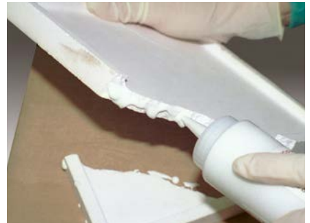
Cerabond™ 503 repairs furnace saggar plate.
