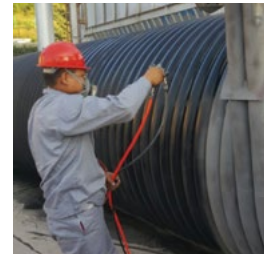
HiE-Coat™ 840-M coats industrial heat exchanger.
