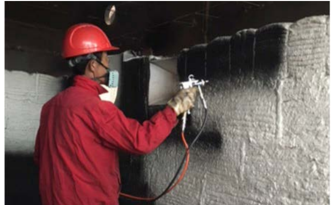
HiE-Coat™ 840-C applied to ceramic fiber module.
