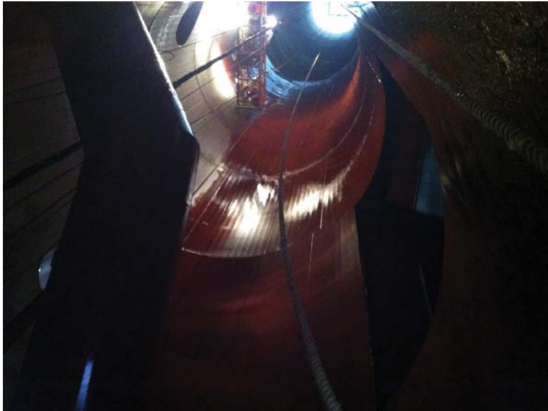
Corr-Paint™ CP2050-LF coats flare stack.
