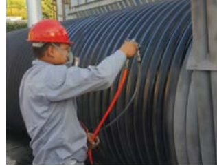
HiE-Coat™ 840-M coats industrial heat exchanger.
