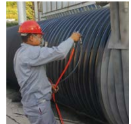
HiE-Coat™ 840-M coats industrial heat exchanger.
